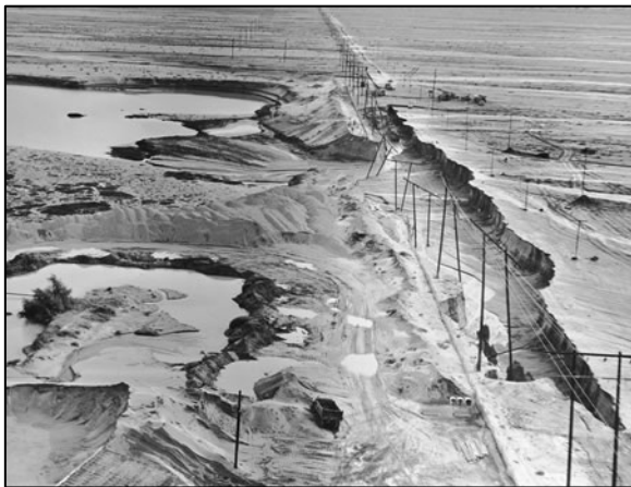
Flood damage to Indian Avenue by the 1965 Whitewater River floodwaters caused the road to be closed for 30 days, adding to the isolation of Palm Springs. (Source: RCFCWCD)
